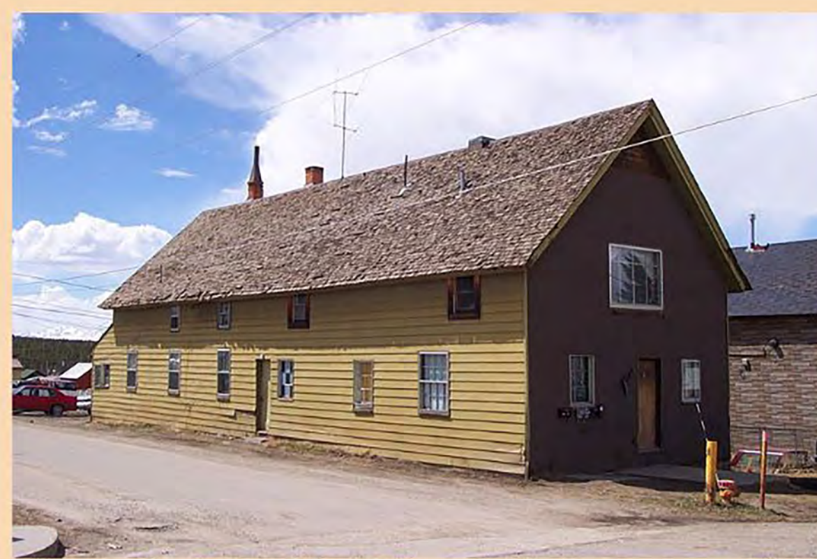
Temple Israel building before restoration efforts began
