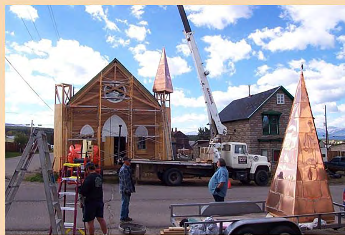
Placement of the copper spires on the front facade
