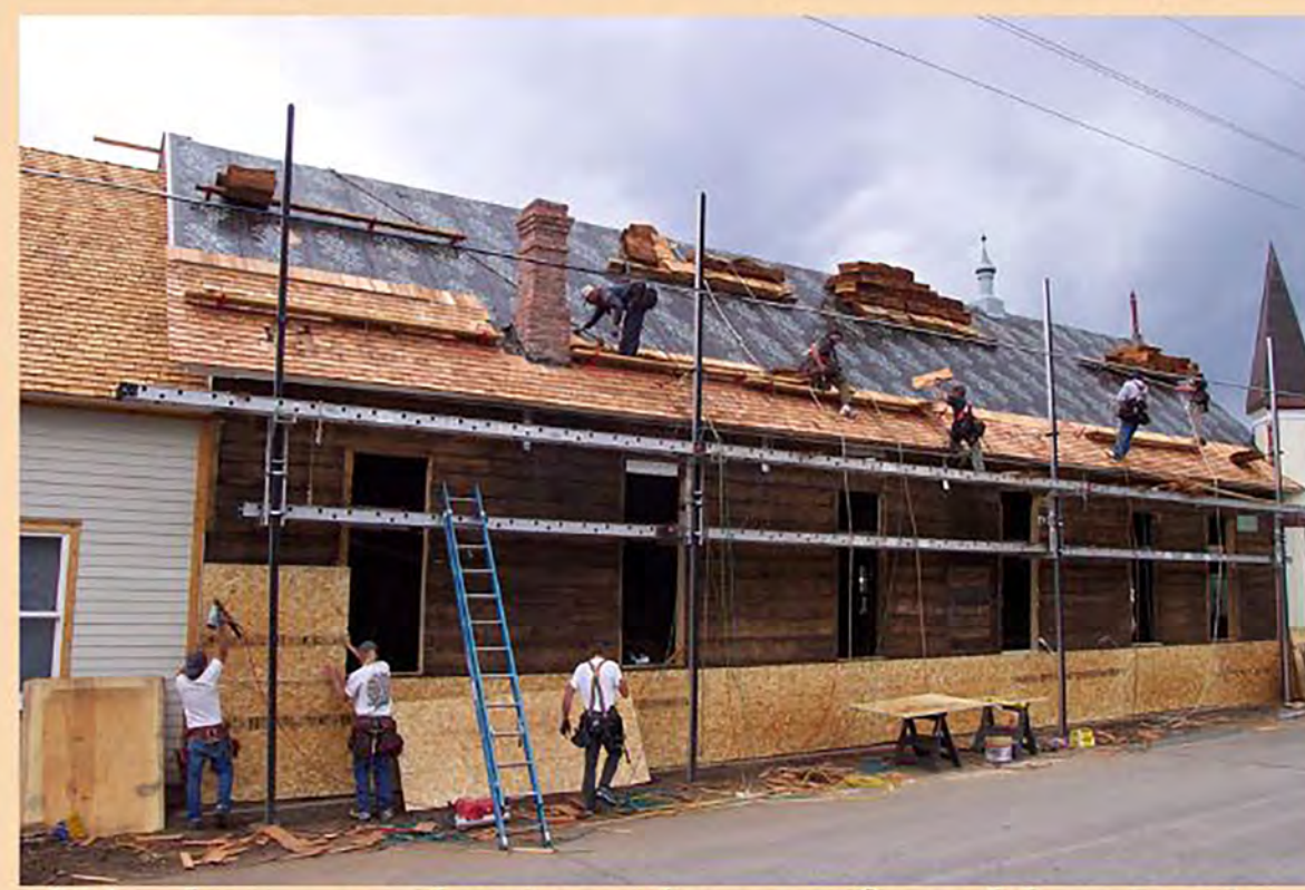
Workers replacing the roof and beginning work on the siding
